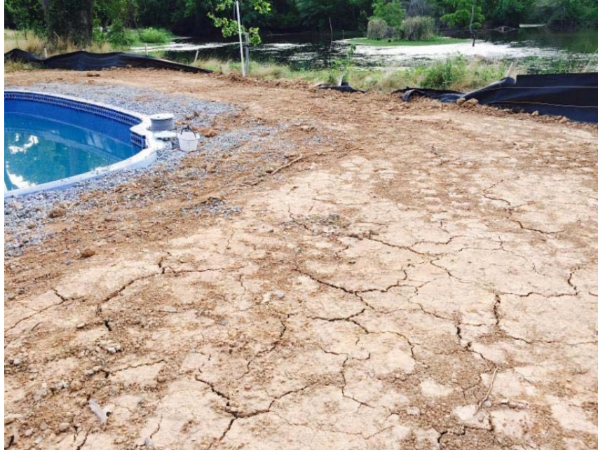
Lack of rainfall caused cracks in the soil on Melinda Ball's property in North Augusta.
