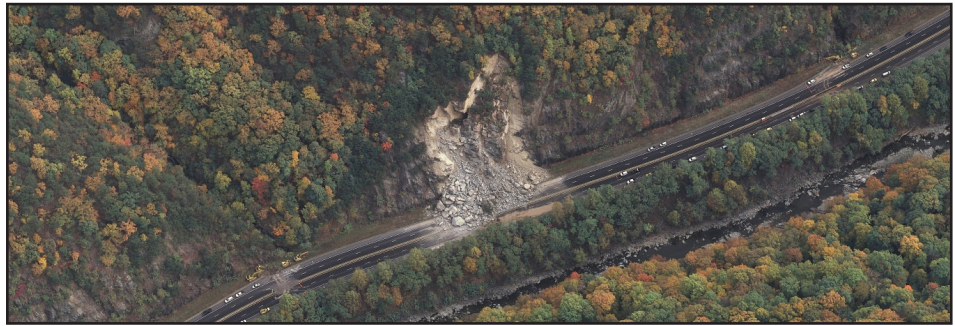
Rock Slide on I-40 in 12/2009 and 01/2012, respectively, in Haywood County near the Tennessee state line. This is the site of repeated rockslides.
