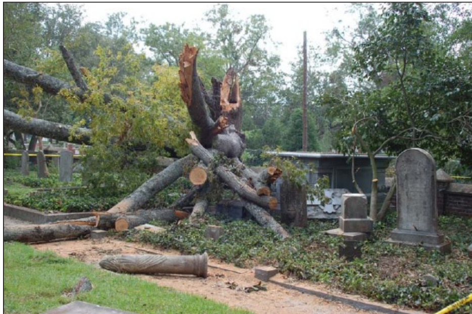
Tree Damage at a Historic Cemetery in Tarboro Resulting from Hurricane Irene, 2011. Photo adapted from Wilds (2011:3).
