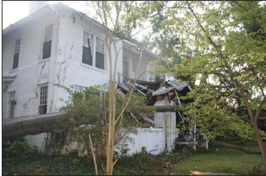
Tree Damage to a National Register Property in Wilson Resulting from Hurricane Irene, 2011. Photo adapted from Wilds (2011:5).
